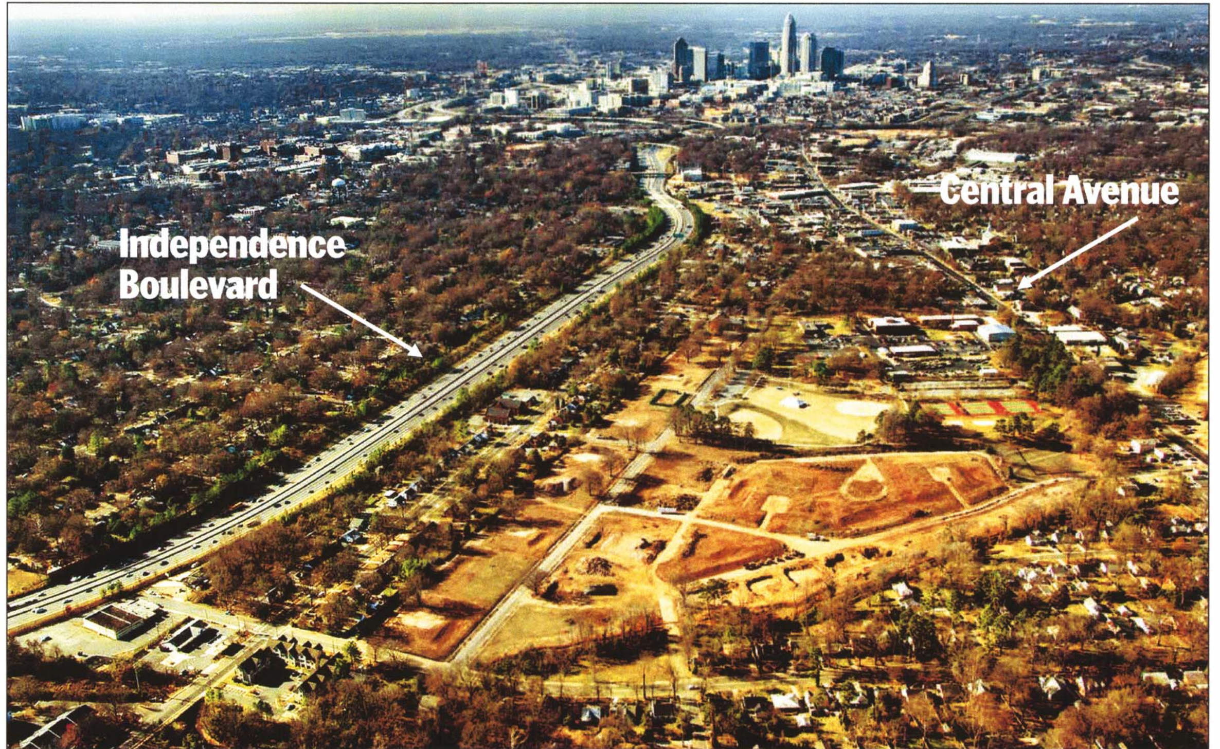
Firmatas LLC demolished Morningside Apartments at McClintock Road and Morningside Drive to clear this 33-acre site for an urban village of residences, shops and restaurants.
